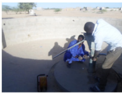
a) Unbolt the casing of the curb.
