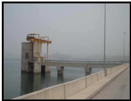
Plate II. Bottom Outlet Structure of Gurara Dam linking transfer pipe to Lower Usuma Dam
